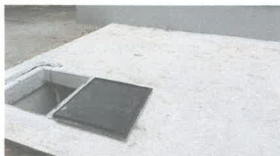
Rainwater Collection Sump3
